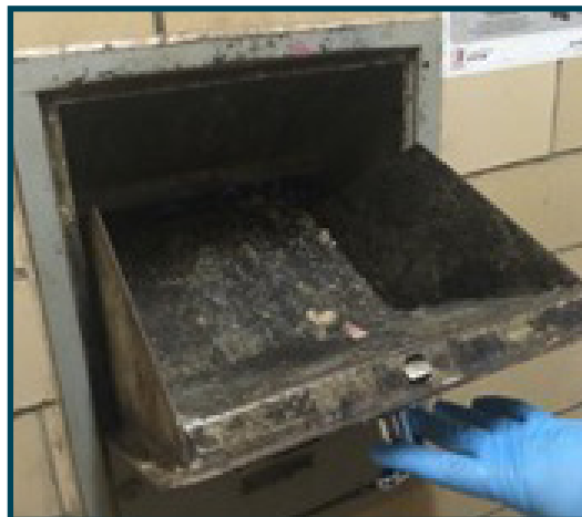
Trash compactor chutes in many buildings are too small to accommodate medium trash.
